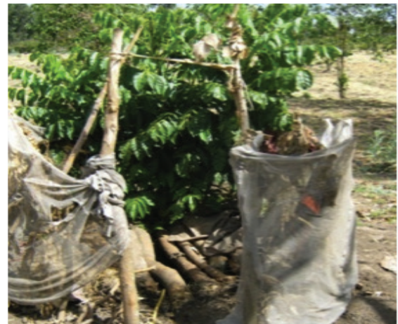
Weak superstructure with lack of privacy
