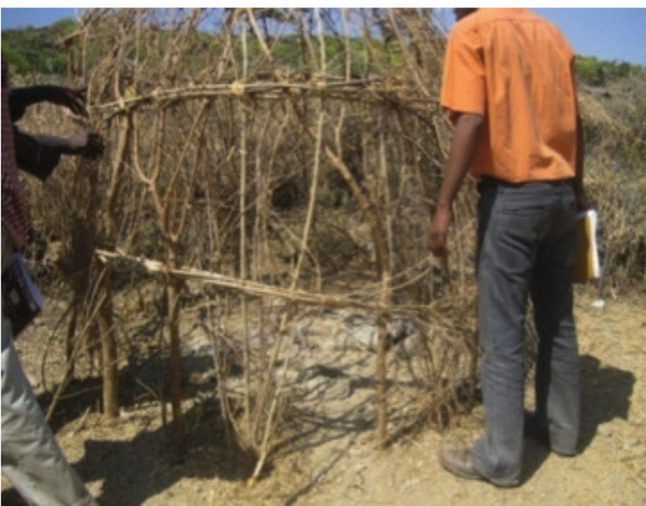
Latrine under construction
