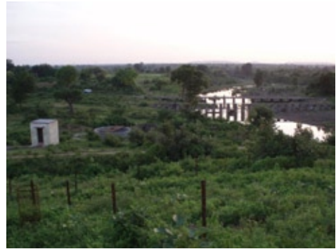
Figure 2: River bank infiltration well in Maharashtra
