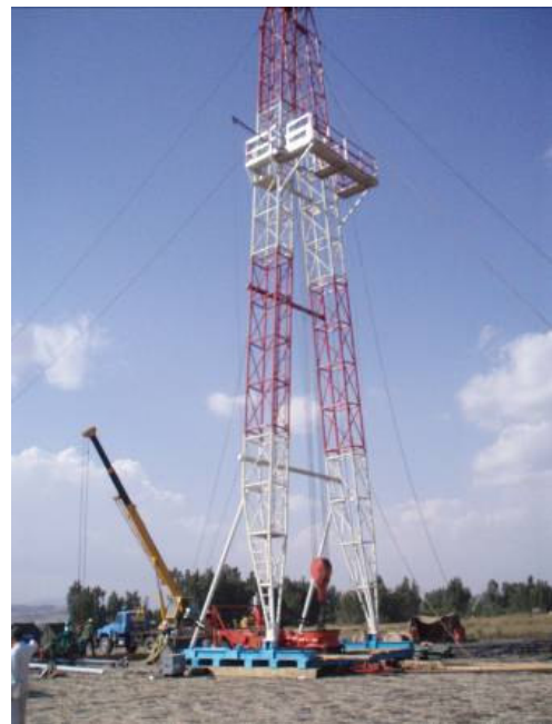
Deep well drilling in Addis Ababa Region
