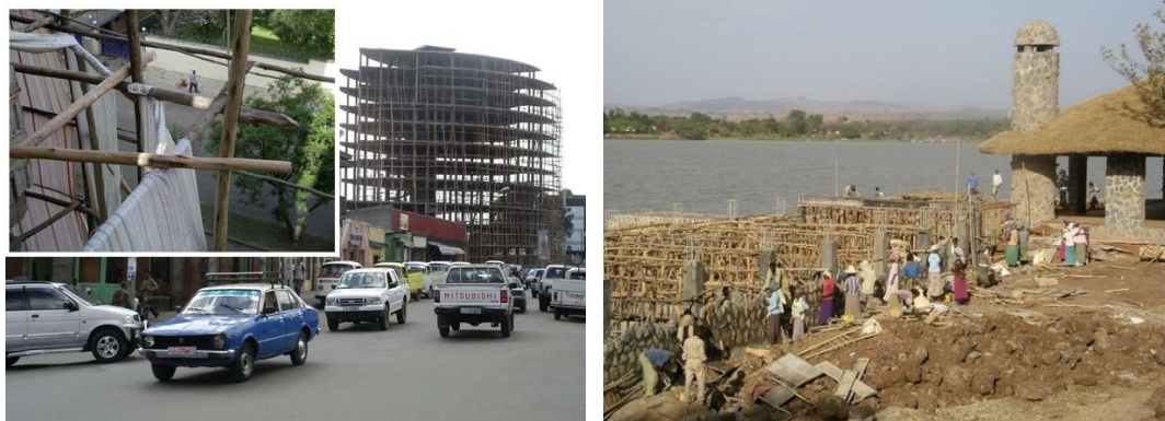
Wood used for scaffolding in Addis Ababa, Ethiopia
