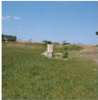
Fanta Spring (chlorination tank)
