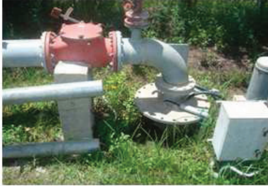
Production well Akaki Wellfield
