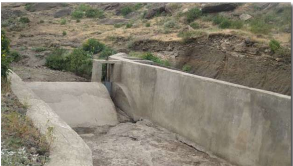
Figure 4 Modern diversion weir in Boru Dodota, Oromia, Ethiopia (Chukalla, 2010).
