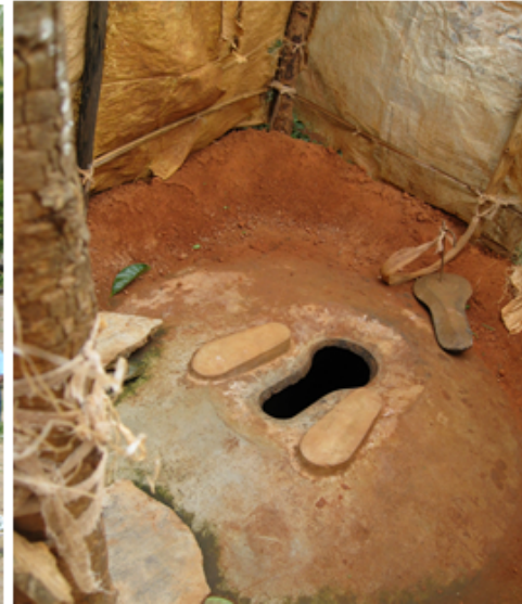
Current scenario - existing squatting pans, common superstructure made of plastic bags and widespread use of open defecation
