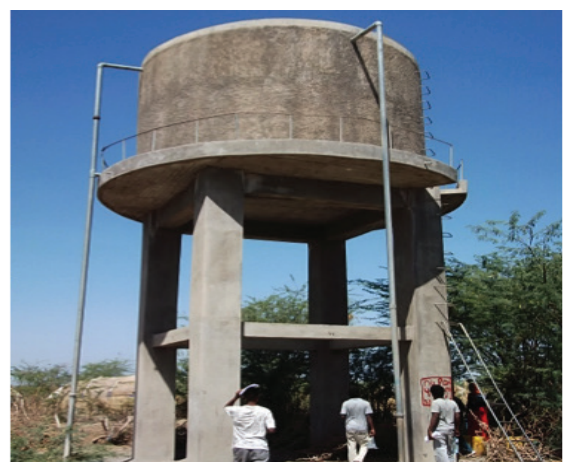
Piped system may have distribution problems
