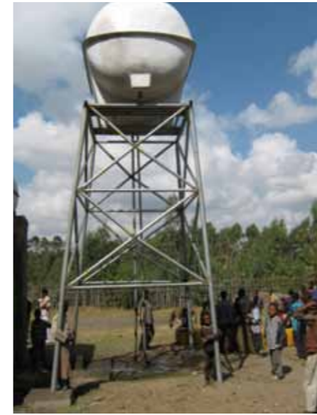
Overhead tank in SNNPR
