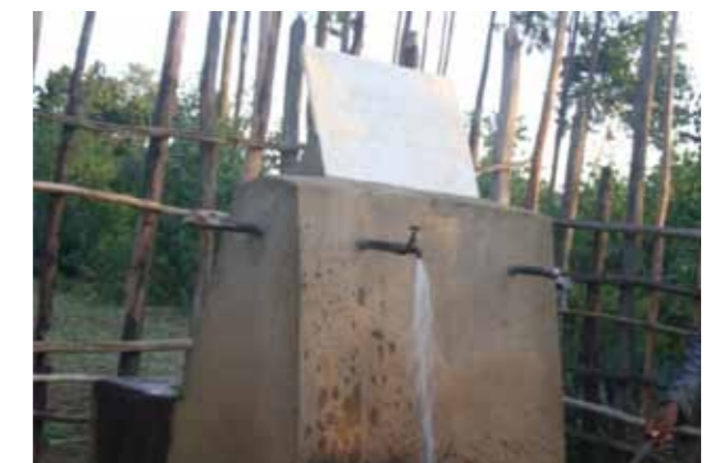
Typical Tap stand in a systems with multiple water points
