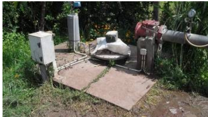
Scope for improving well head protection
