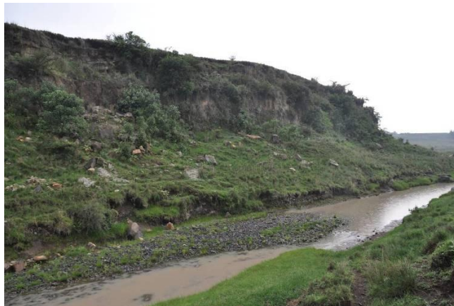
The right embankment at the proposed axis. The rock can be seen.
