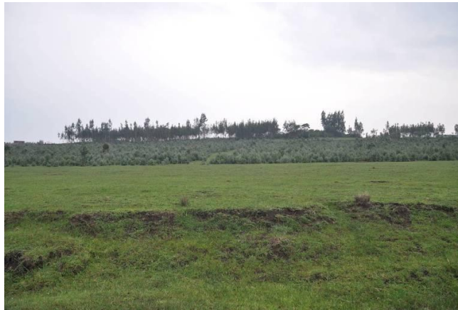
The left embankment on the proposed axis.
