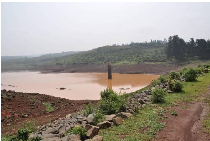
The Geffersa III dam with the new tower intake
