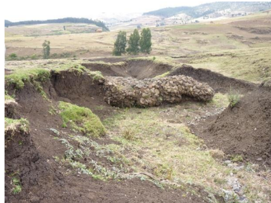
Figure 15: Badly positioned gabion gully plug (Dire)
